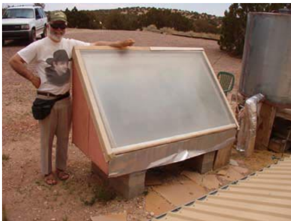
Front View, Kerr-Cole Main Solar Water Heater
